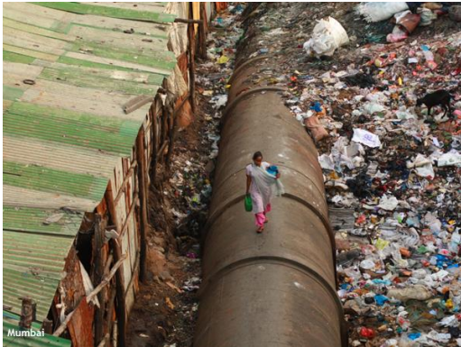
Mumbai water supply without access for the poor
