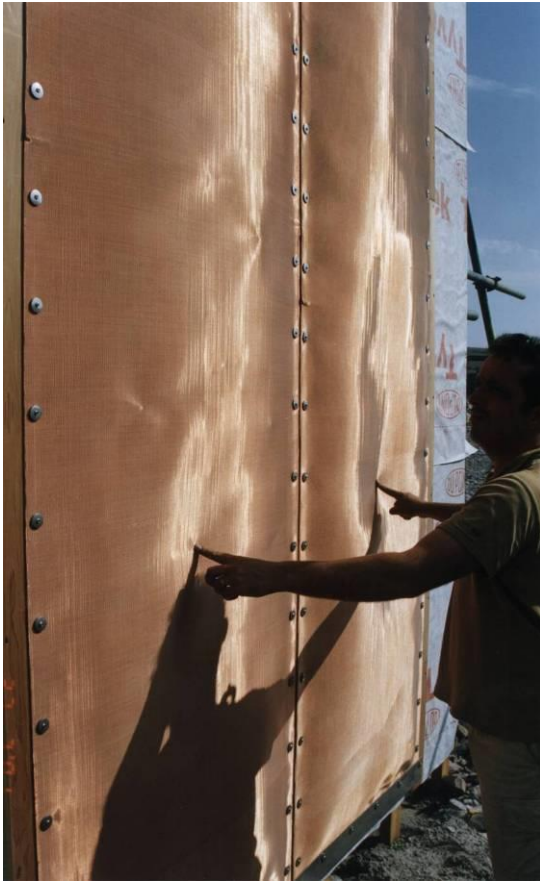
Image: woven phosphor bronze wire cladding - soft metal jacket
