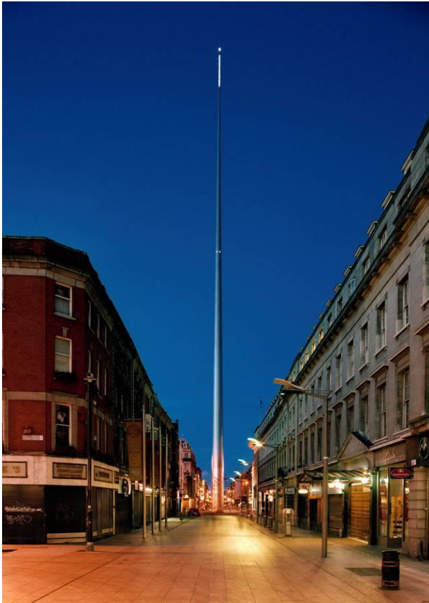
Image: Conical shell of 3m dia. base, 120m high, made of shot-peened stainless steel plate International competition winners 1998.
