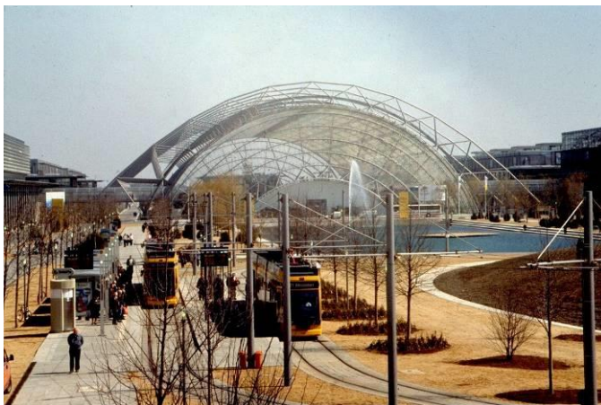
Image: 25,000m 2 of internally suspended colourless laminated glass vault, 250m long, 80m clear span and 30m high. The glass is cleaned externally by 2 robots driven from the apex of the roof. Leipzig Glass Hall, Ian Ritchie Architects with gmp and Mero-Seele JV, 1993-96
