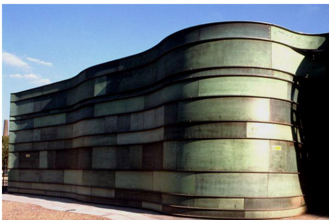
Image: Culling Road: 'I saw a hundred greens in the grass in Southwark Park' Multi-green post-patinated copper sheet cladding.
