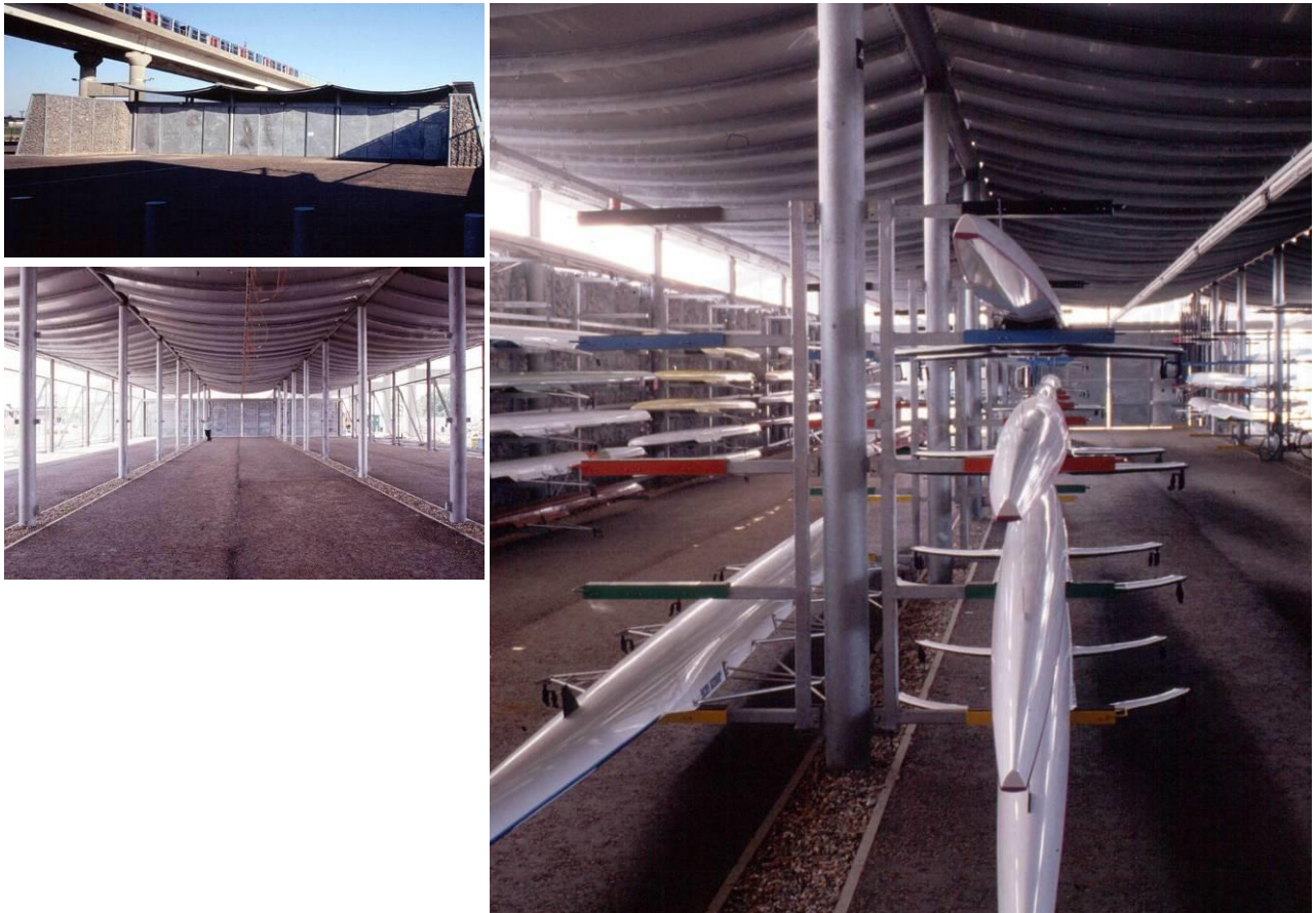
Image: Stone filled gabion ; stainless steel sheet catenary roof London Intl. Regatta Centre, Ian Ritchie Architects with Arup, 1994-98
