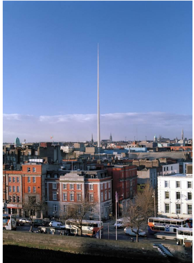
Image: Conical shell of 3m dia. base, 120m high, made of shot-peened stainless steel plate International competition winners 1998.
