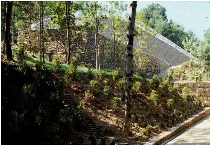
Image: Gabion walls as architectural enclosure helping to create the building's own micro-climate solely through solar energy and evaporative cooling. Jardin de L'imaginaire landscape, K Gustafson. Terrasson Cultural Greenhouse, Ian Ritchie Architects with Arup, France Gabion, Glasbau Seele, 1992
