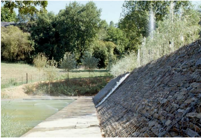
Image: Gabion walls as landscape architectural retention walls.
