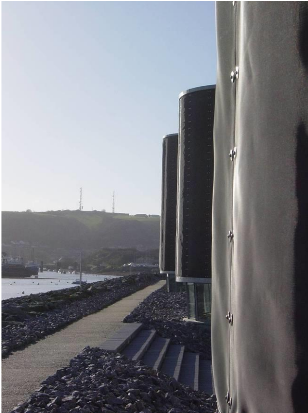
Image: Soft woven phosphor bronze wire cladding
