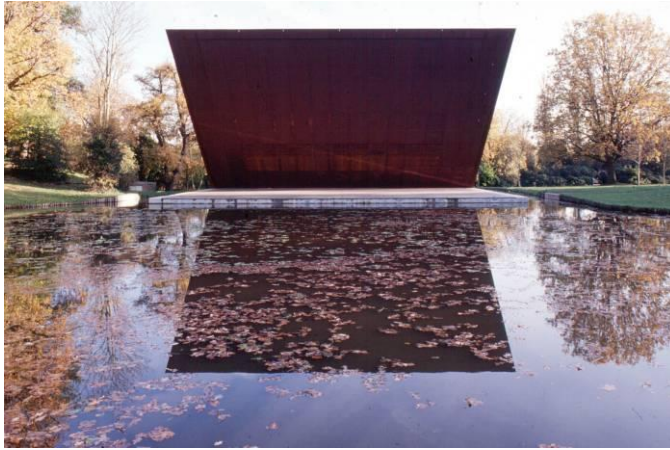
Image: Concert Platform: Zero-maintenance project using Corten A oxidised steel and oak, with integrated 'LARIS active acoustic system'. Competition winners 1997.
